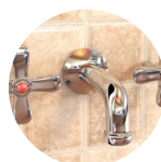
All Plumbing & Bathroom Pipes
